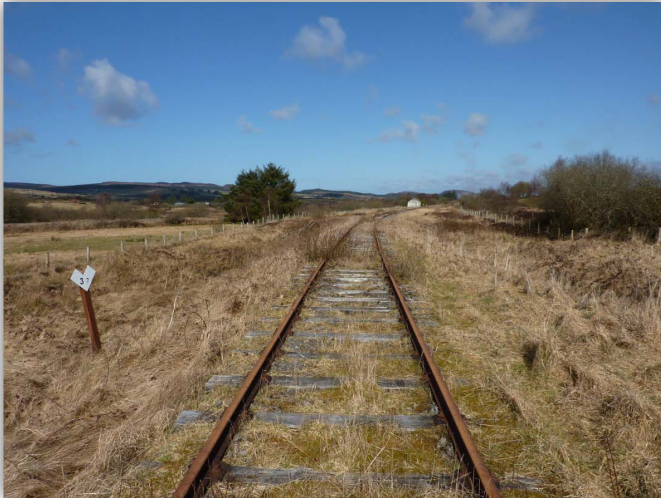
Photo 13 Looking Northeast towards Carrowloughan (copyright West=on=Track)
