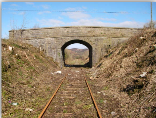
Photo 9 Railway Overbridge (copyright West-on=Track)
