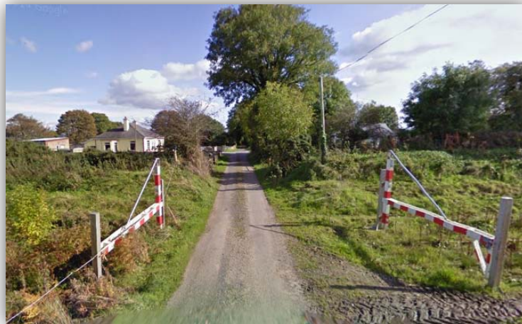
Photo 12 Level Crossing at Curry South (source: google.ie)
