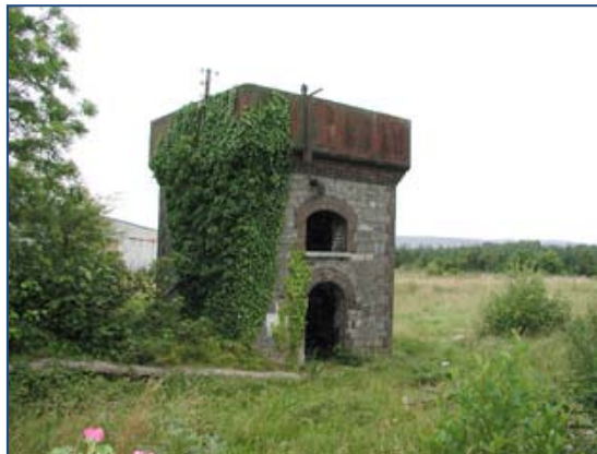
Water Tower at Tubbercurry (source: NIAH)
