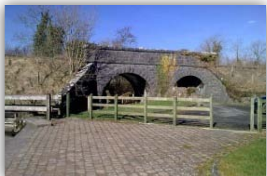
Photo 5 Underbridge at Curry (source: sligotrails.ie)
